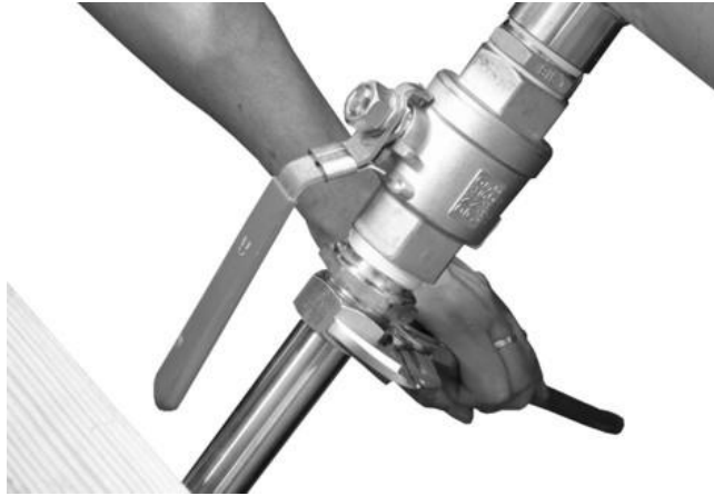
Fig. 10-33 Fastening the sensor
