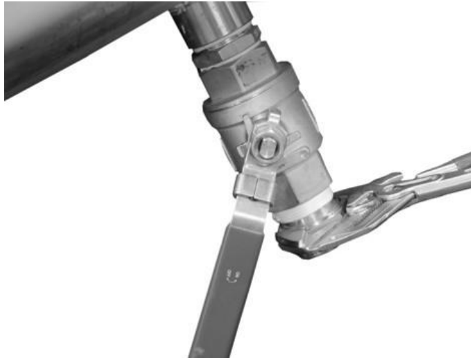
Fig. 10-31 Fastening the sensor screw connection to the ball valve
