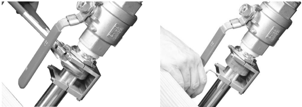
Fig. 10-39 Secure sensor again during installation
